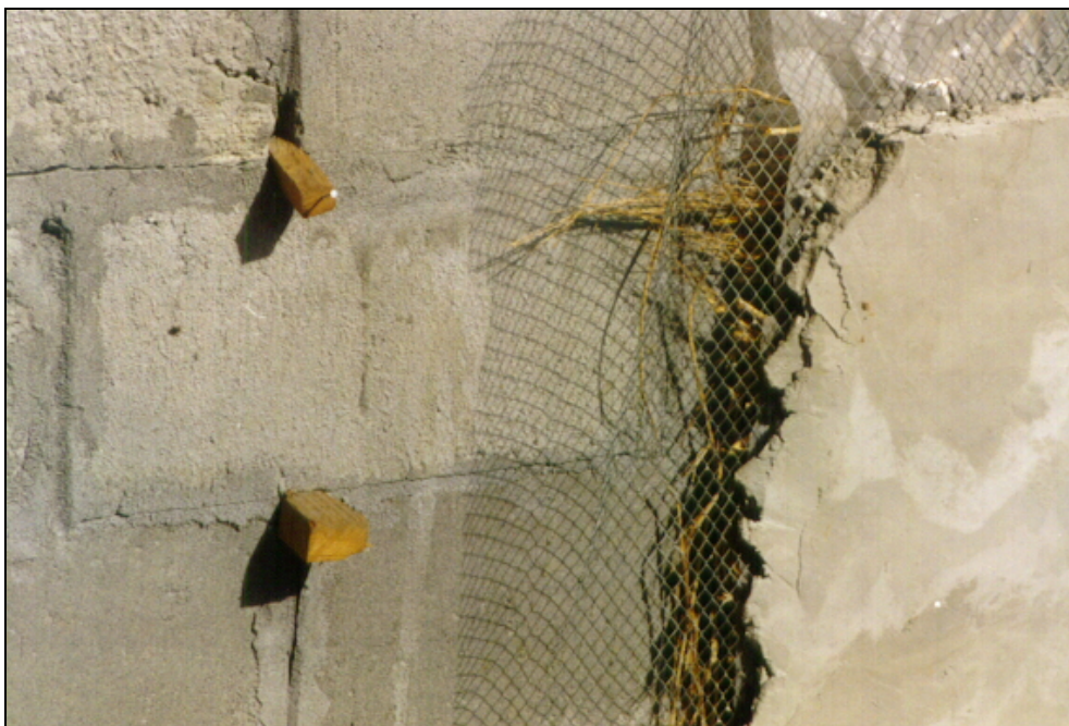
FIGURE 19. PEGS MASONED INTO THE WALL FOR ATTACHMENT OF PLASTIC AND EXPANDED METAL.
