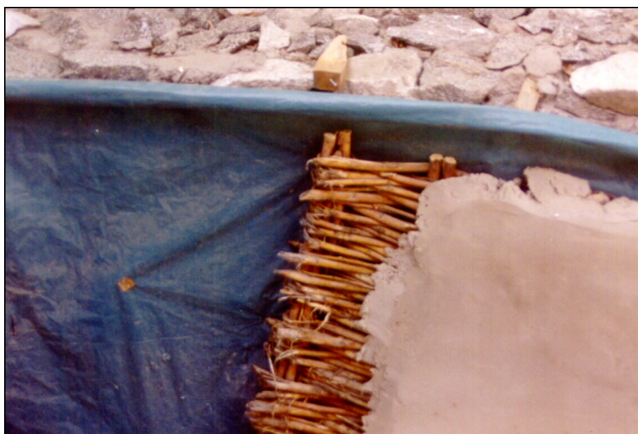
FIGURE 15. CAVITY WALL WITH WATTLE PANEL (THIS WALL IS NOT FINISHED ABOVE THE PLASTIC)
