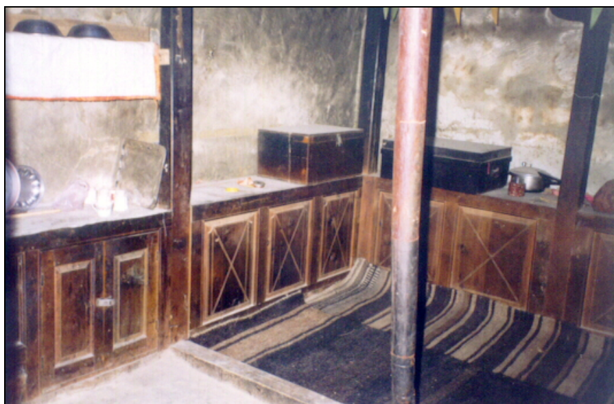
FIGURE 14. WOODEN GRAIN STORAGE BOXES AGAINST THE WALL ARE EXCELLENT INSULATORS
