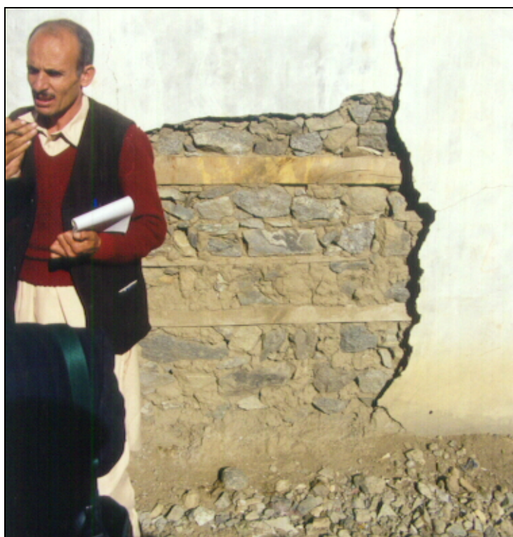
FIGURE 3. CEMENT PLASTER (WITHOUT EXPANDED METAL) WILL EASILY BREAK OFF STONE WALLS
