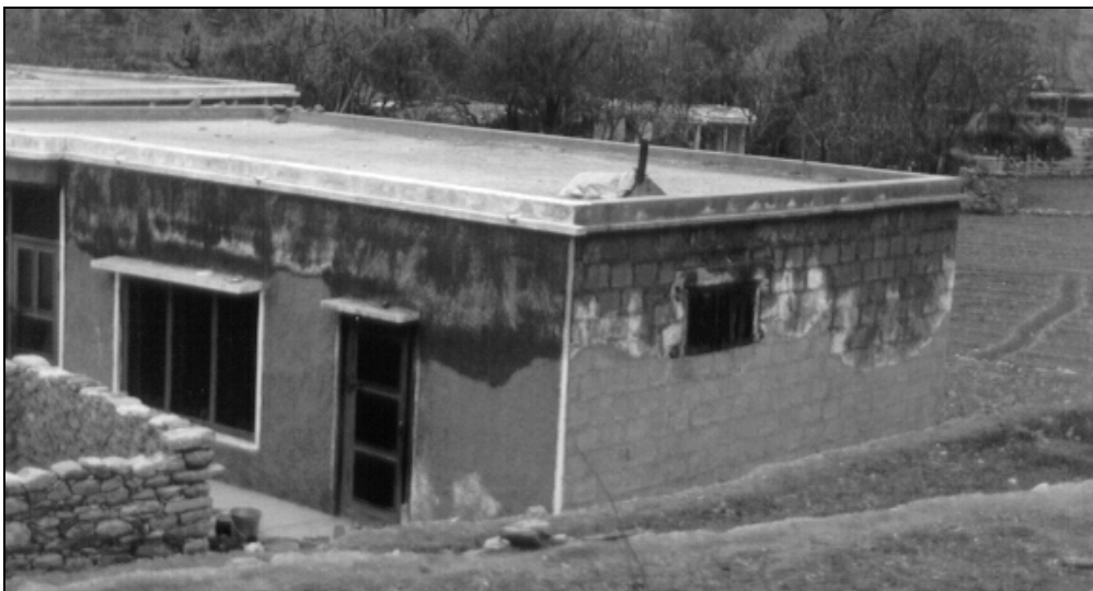
FIGURE 10. WET WALLS (FROM FOUNDATION OR ROOF) NEED TO BE TREATED SO THEY BECOME DRY
