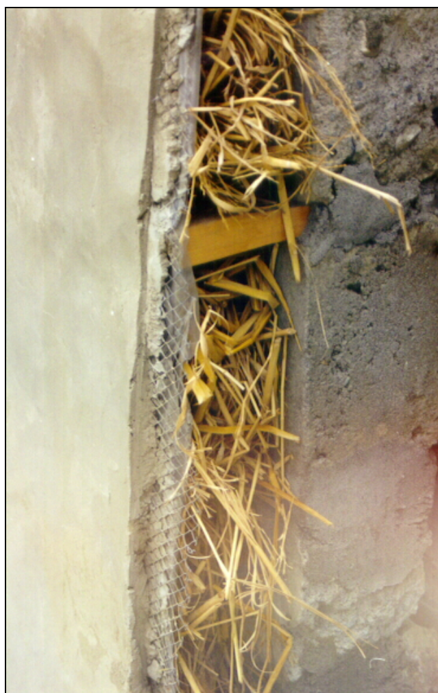
FIGURE 12. CEMENT BLOCK WALL WITH STRAW INSULATION AND PLASTE
