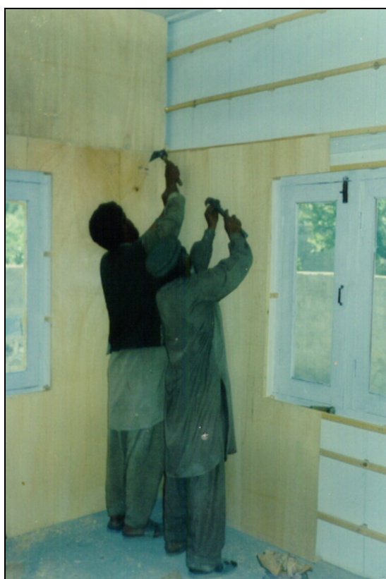
FIGURE 21. APPLICATION OF 1/8" PLYWOOD ON EXISTING CEMENT BLOCK WALL CREATING AIR INSULATION
