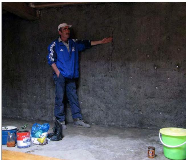
The construction in the above picture is made from the thick sheep wool backed with reflective foil, a space, common plastic foil (0.1 or 0.2 mm recycled), fine wire-mesh and plastered with cement plaster. The picture is made after the first cement plaster coat. A second cement plaster and lime coat will provide a smooth and durable finish. A plinth, white washing or wallpaper will finish the job, according to the liking of the house owner.
