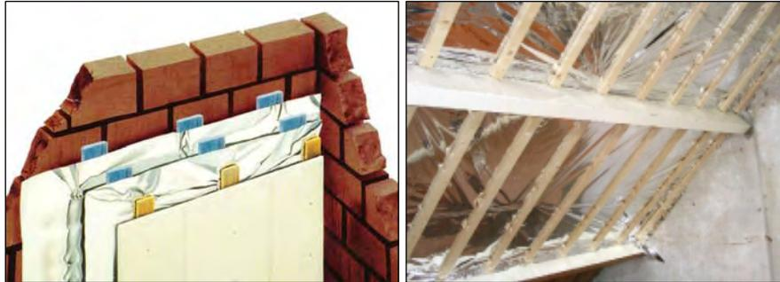
Far Right: 2 reflective foils on 2.5 cm strips against an inclined construction such as a roof; not yet covered.
