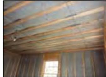
The thickness of sheep wool blankets can vary from a thin 5 cm to 20 cm thickness. Wool is a nice material to work with. The batts (sheets) are held together with 12% polyester.
