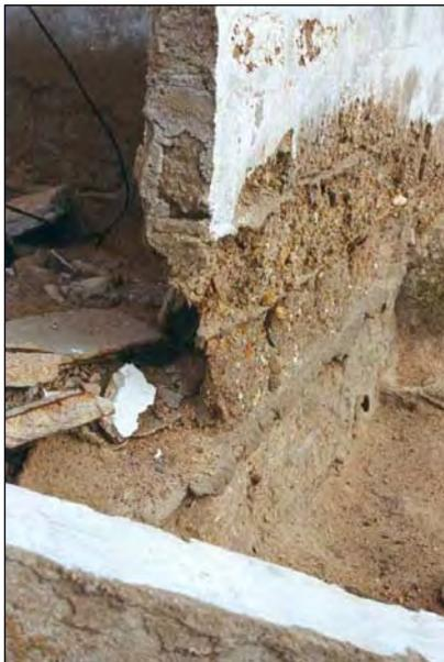
Rising moisture from the soil and then evaporation in dry weather may cause crystallization of the mineral and salts in the water, which will cause damage to the surface of the wall and result in erosion of the wall construction as can be seen in the left picture.
