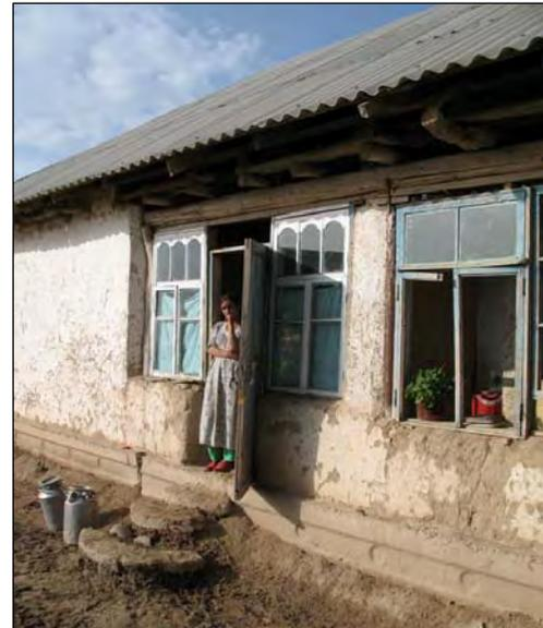
Both adobe blocks and rammed earth walls are hygroscopic materials and have high moisture absorption characteristics. A benefit is that the hygroscopic characteristic of adobe and clay-soil construction materials helps to stabilize the possible air humidity fluctuations inside the house, improving inside climate.
