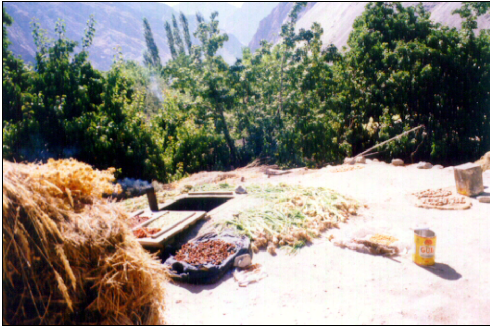
Typical situation where the roof is used for stacking hay and drying fruit. The wooden plank is used to close the roof hatch in the event of severe cold or rain. The chimney is sticking out of the hole.
