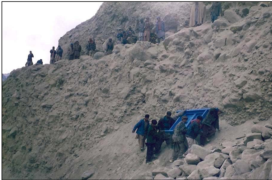
TRANSPORT OF A LARGE BUILDING COMPONENT ACROSS A LANDSLIDE
