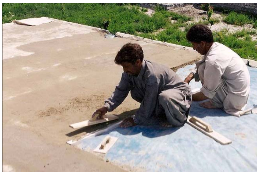
APPLYING WATERPROOFING AND PROTECTION OVER AN INSULATION LAYER
