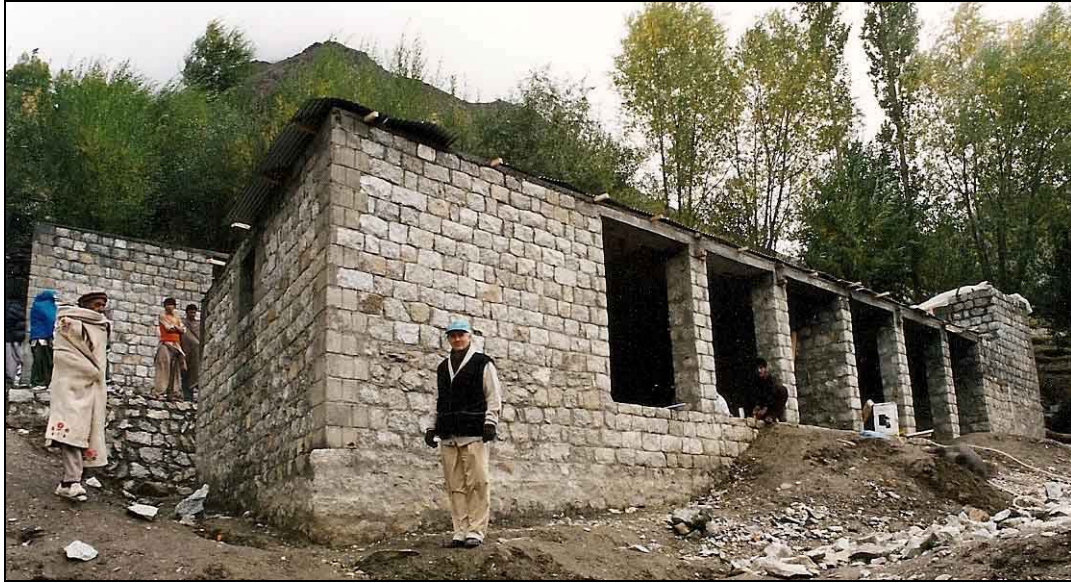
FRONT BUILDING OF GARTENZ SCHOOL IN PROGRESS OF CONSTRUCTION LARGE WINDOWS ON THE SUN SIDE, STOREROOM ON LEFT END FACING COLD VALLEY WIND, AND TOILET BLOCK ON RIGHT END
