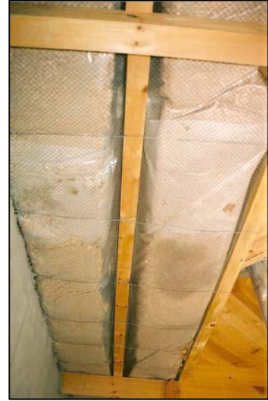
CEILING WITH INSULATION MATERIAL BEFORE FIXING THE SUSPENDED CEILING
