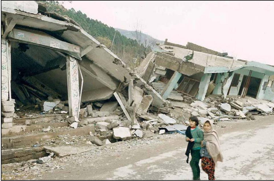
HEAVY CONCRETE FLOORS AND FAULTY DESIGN OF TOP AND BOTTOM COLUMN REINFORCEMENT CAUSE COLLAPSE
