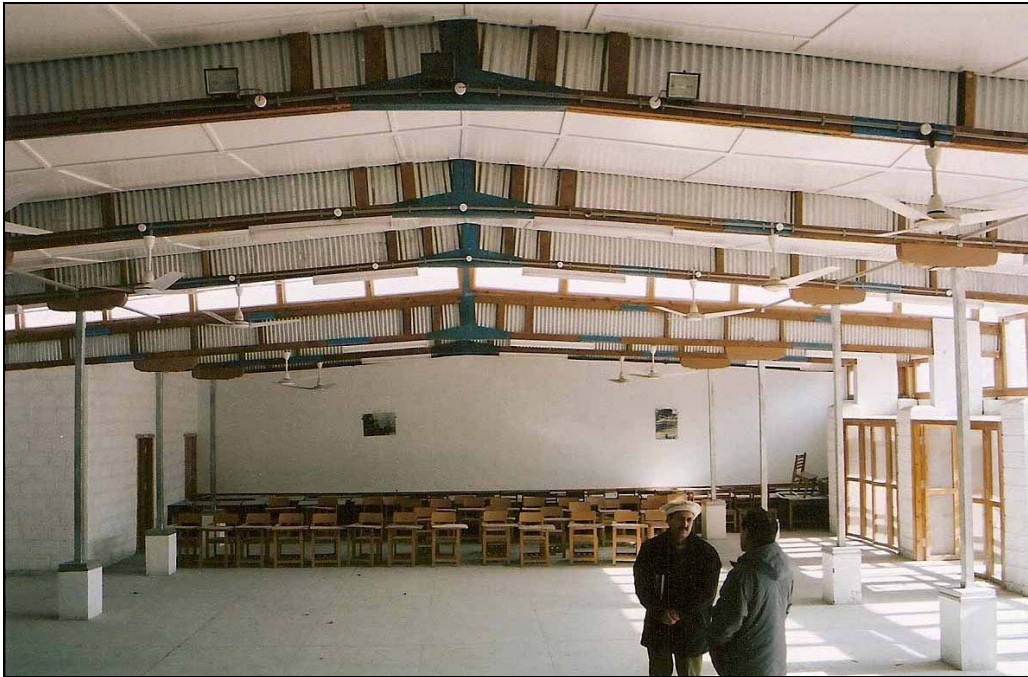
ESPECIALLY DESIGNED LONG SPAN COMPOSITE BEAMS FOR THE AL AZAR EXAMINATION HALL
