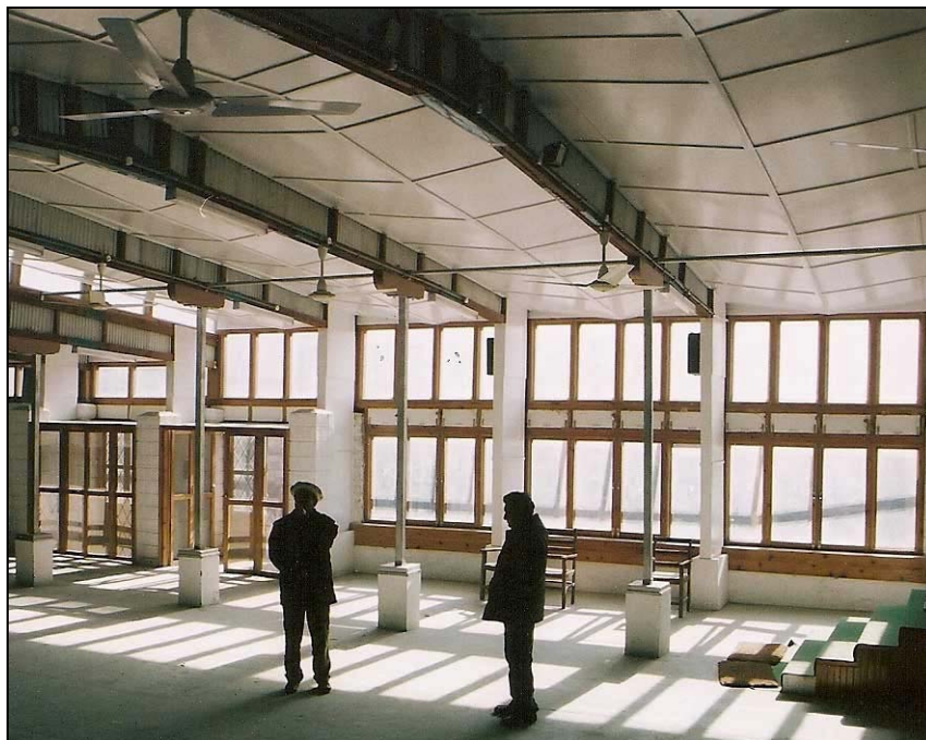
THE AL AZAR EXAMINATION HALL INCLUDED SEVERAL COMPONENTS EXPLAINED IN THIS REPORT: SOLAR WINDOWS, THERMAL WALL AND ROOF INSULATION, COMPOSITE AND BOWSTRING BEAMS
