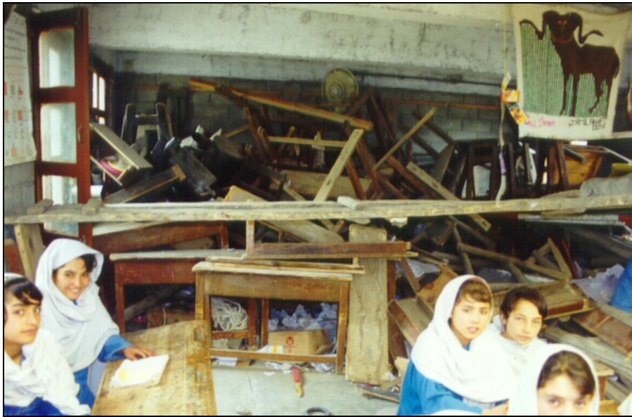
PILED-UP BROKEN FURNITURE IN THE BACK OF A CLASSROOM
