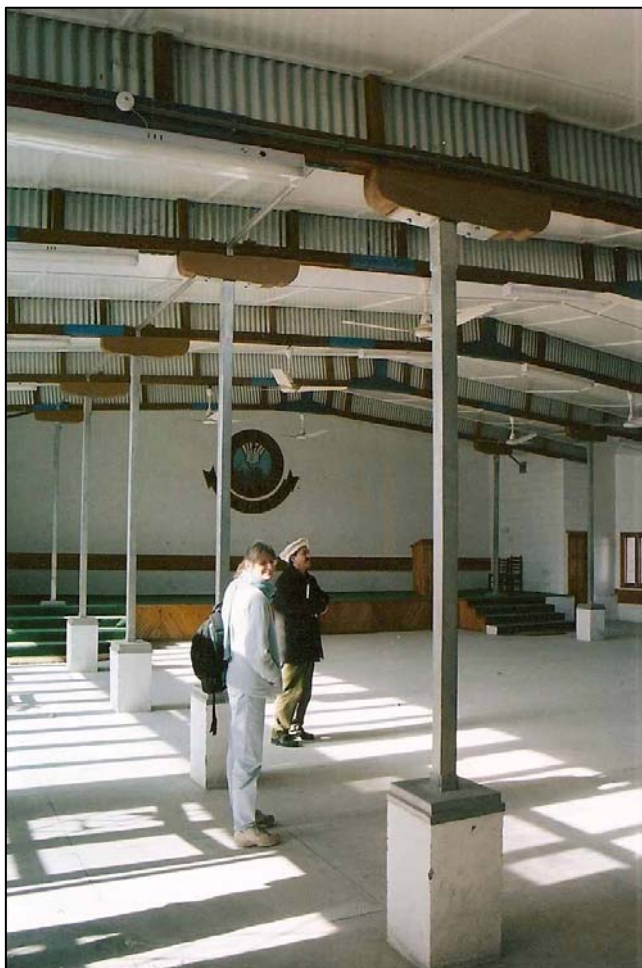
SLENDER COLUMNS WITH LARGE SPAN COMPOSITE BEAMS THESE 3.5" x 3.5" COLUMNS CAUSE MINIMAL VISUAL OBSTRUCTION THE TABLE-HEIGHT CONCRETE COLUMN REDUCES THE BUCKLE LENGTH
