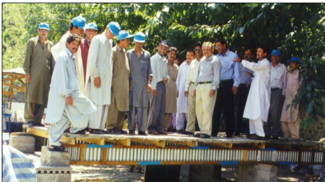
TESTING OF A THIN, LIGHTWEIGHT STRONG FLOOR FOR SHORT SPAN CONSTRUCTIONS
