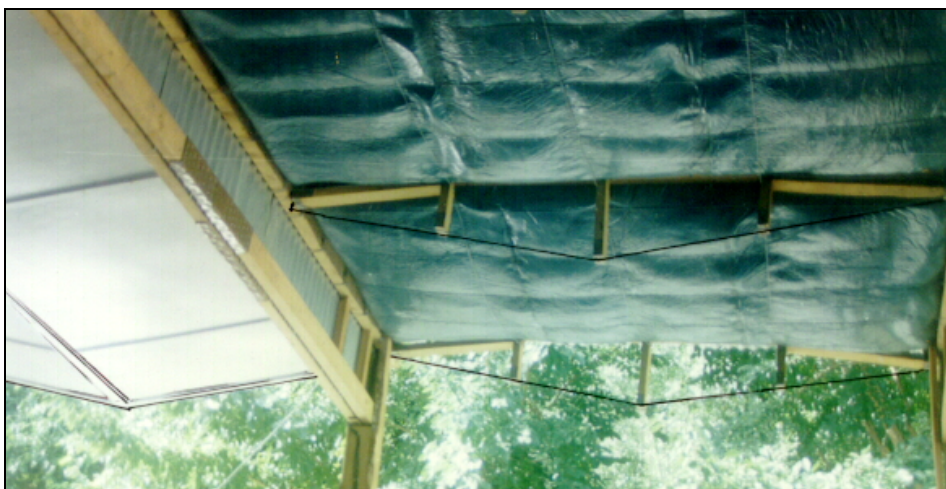
COMPOSITE SUPPORT BEAMS WITH BOWSTRING BEAM REALISATION OF INSULATION AND SUSPENDED CEILING UNDER GI ROOF
