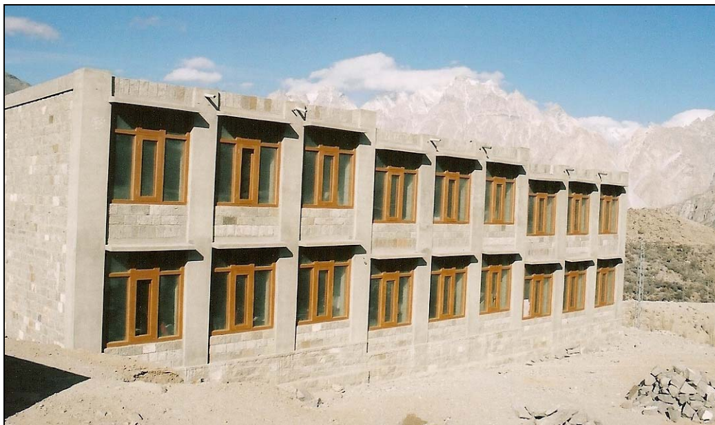
GHULKIN SCHOOL NEW FAÇADE WITH MODIFIED WINDOW FRAMES
