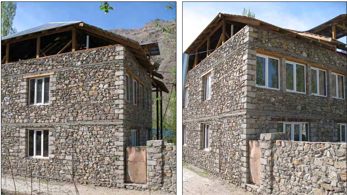
A house masoned with wire-mesh reinforcement and corner L- and U-shaped cement blocks used. The cement blocks allow fast construction of straight corners of the walls and straight sides along the windows. In a later phase, the house owner can plaster the walls.
