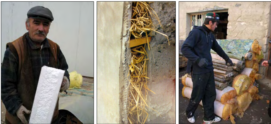
Expanded Polystyrene (EPS) and glass wool insulate twice as good as straw for the same thickness. Low quality and compressed glass wool has a lower insulation value than EPS per same thickness. Straw is usually much cheaper than EPS, but can be affected by moisture and insects. The entrepreneur should be able to explain the cost and use differences to their clients.
