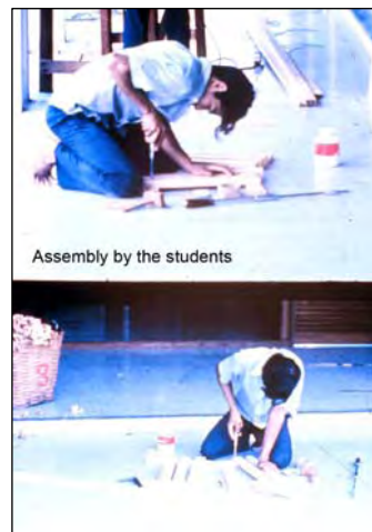
Construction is simple. All timber is the same thickness and width and only two widths are used.
