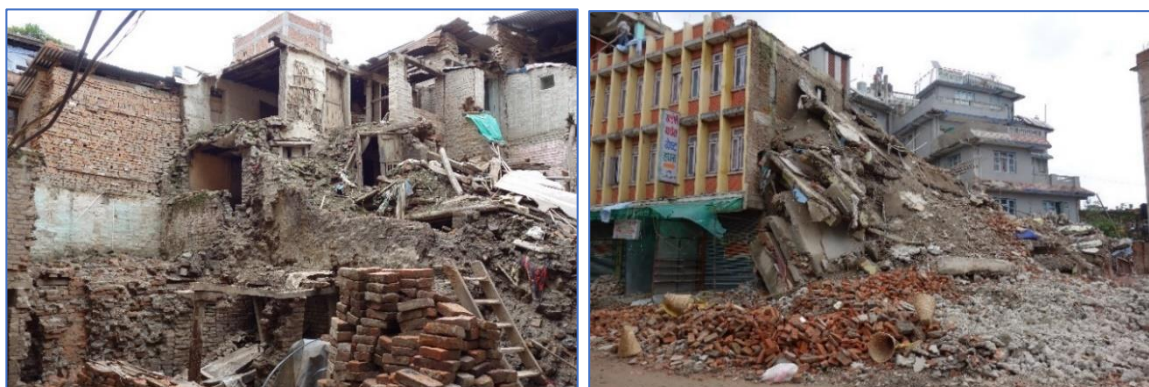
Figuren 86. Ingestorte woningen in Kathmandu stad 2015. (E.f.).
