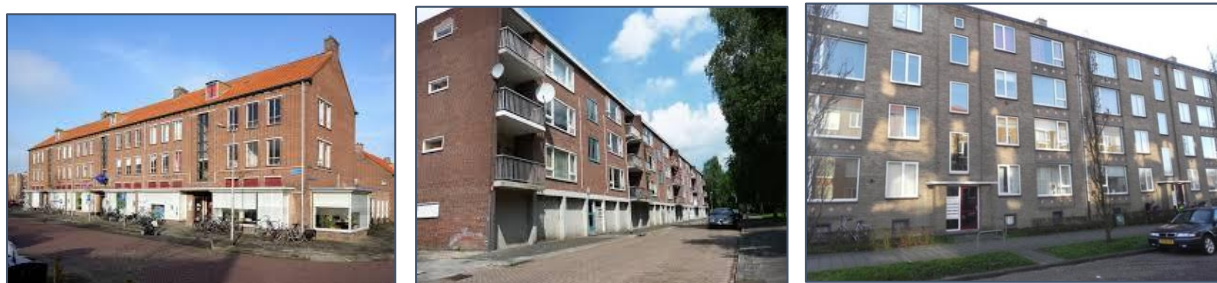
Figures 65. Left: CC1B, three floors. Middle: CC1B three floors. Right: CC2, four floors In the middle picture there are four floors, but the bottom floor is not inhabited (garage boxes), therefor only three floors apply with CC1B qualification.
