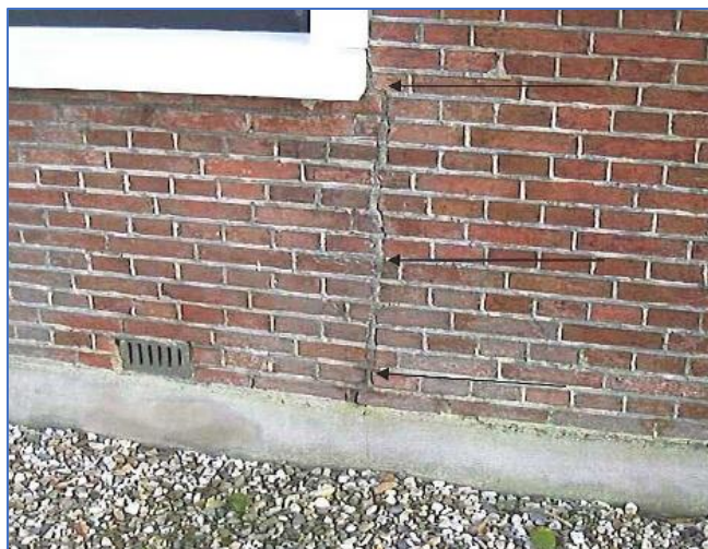
Figures 63. Numerous cracks arise from the foundation due to small settlements in foundations on solid ground. These cracks extend to the window openings on the ground floor. These are very common even without earthquakes, especially in brick buildings with cellars. These cracks are aggravated by (earthquake, traffic) vibrations.
