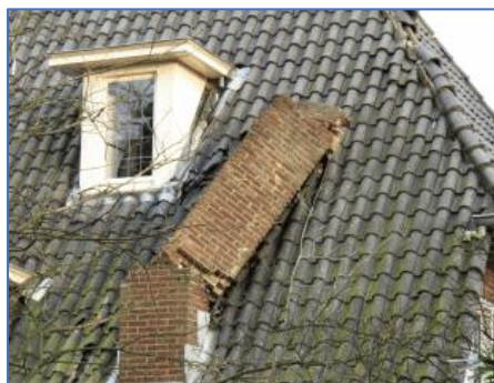
Figures 59. High-risk elements include heavy chimneys on a flexible timber roof structure, balconies wedged into brick walls, and spandrels or free-standing gable ends that sit on buildings and above sidewalks. While falling, they can cause casualties in the public space. Middle and right. Building with high-risk elements: heavy chimney on a weak roof, wedged cantilevered balcony (red), and a building without these high-risk elements (blue). 81
