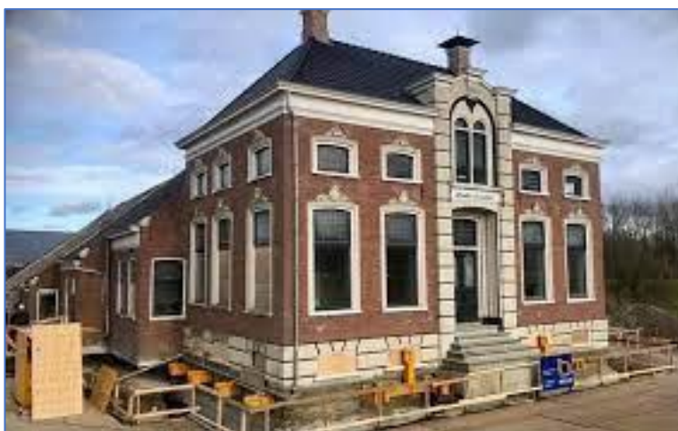
Figure 63. At this historic end house of this farm in Garrelsweer, cracks appeared in the foundation and basement in 2006 and 2012 due to the earthquakes. In combination with the already occurring land subsidence and the resulting increased groundwater level, the groundwater ran into the basement.
