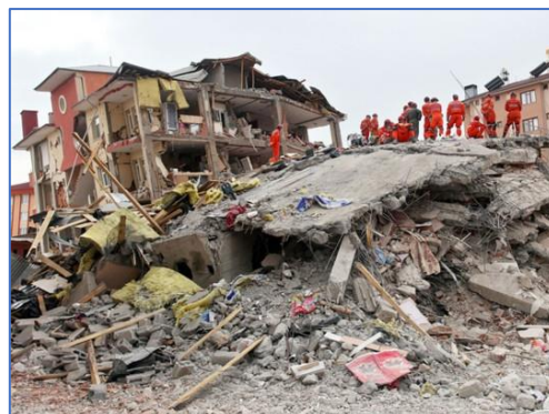
Figures 25. Left. The wrong design/situation with ridged floors and flexible columns (red.) Middle. Good design/situation with strong columns and flexible floors (blue). Right photo. With the failure of columns, the entire building will collapse, and the building will pancake.
