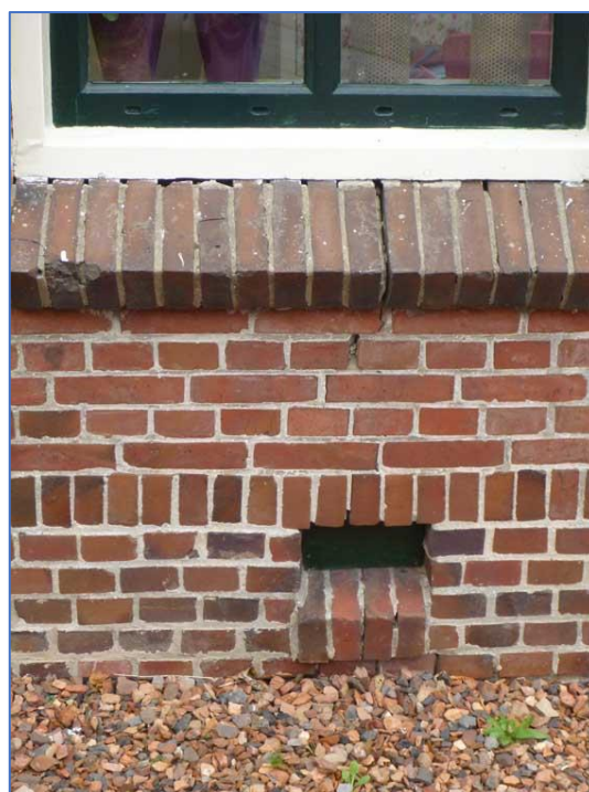
Figures 63. Numerous cracks arise from the foundation due to small settlements in foundations on solid ground. These cracks extend to the window openings on the ground floor. These are very common even without earthquakes, especially in brick buildings with cellars. These cracks are aggravated by (earthquake, traffic) vibrations.
