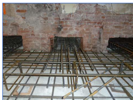
Figures 56. Photo and sketch of the construction of a platform foundation in an existing building. By making a fully load-bearing plate under the entire building, the ground pressure is reduced even more. See also Chapter 4.
