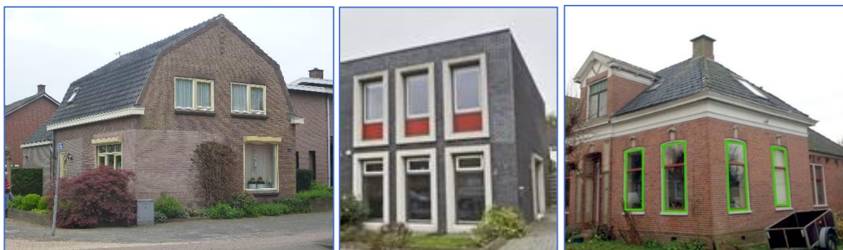
Figures 92. Left. Masoned-up window Middle. Strong window edges Right. Constructive Glass panels
