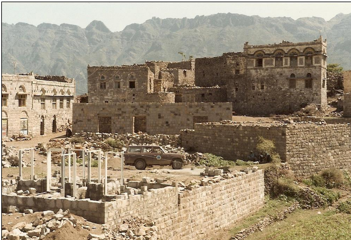
RECONSTRUCTION ON AN EXISTING PLOT IN A VILLAGE. THE MASONED RETAINING WALL WAS CONSIDERED ADEQUATELY STRONG ENOUGH FOR THE NEW ONE-STOREY HOUSE. AFTER THE RECENT EARTHQUAKE, THE WALL DID NOT SHOW ANY DAMAGE.
