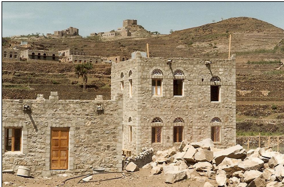
NEW CONSTRUCTION TECHNOLOGY REALIZED BY THE SELF-HELP RECONSTRUCTION PROJECT
