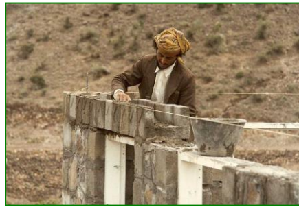
Local masons first placed the U shaped cement blocks after which the dressed stones were masoned in cement mortar and reinforcements.
