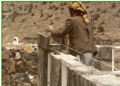
Local masons first placed the U shaped cement blocks after which the dressed stones were masoned in cement mortar and reinforcements.
