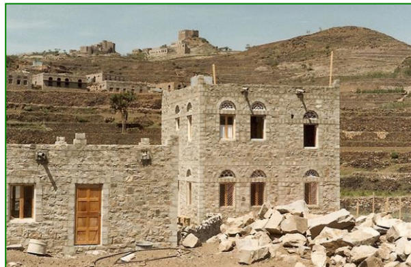
Local masons first placed the U shaped cement blocks after which the dressed stones were masoned in cement mortar and reinforcements.
