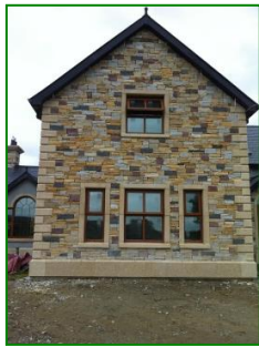
Houses in Britain with straight tailored cornerstones, providing a distinctive architectural feature.
