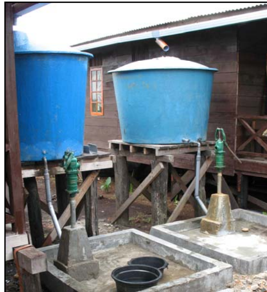
RAINWATER HARVESTING COMPLEMENTED WITH A SHALLOW WELL FOR WASHING WATER
