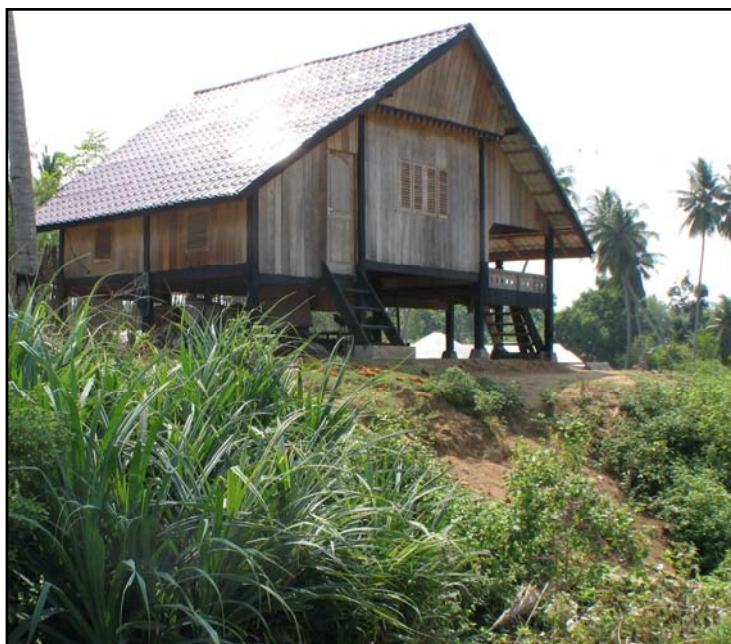
GOOD EXAMPLE OF A NEW TIMBER HOUSE – BUILT FARTHER AWAY FROM THE SEA, ON A HILL AND ON SHORT STILTS. THE ROOF IS LIGHTWEIGHT METAL AND THE OWNER HAS APPLIED WOOD PRESERVATIVE ON THE STRUCTURAL MEMBERS.
