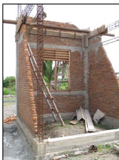
DEMONSTRATION UNIT ON CONSTRUCTION
