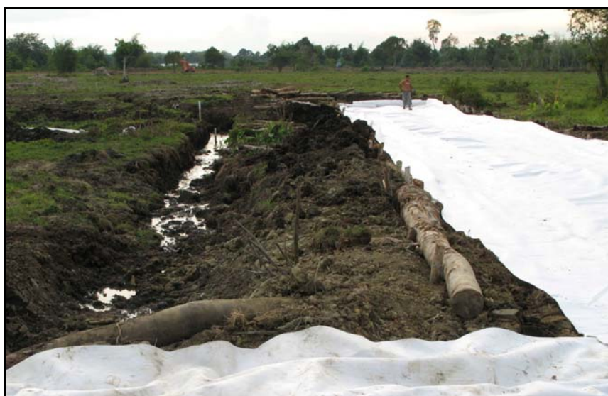
LAYING OF A ROAD FOUNDATION CLOTH ON SWAMPY SOIL BY THE NGO
