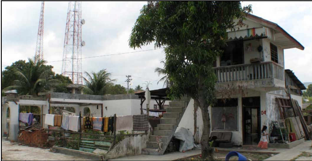
THE GROUND-FLOOR-ONLY HOUSES WERE DESTROYED BUT THE SECOND STOREY OF THIS HOUSE SURVIVED
