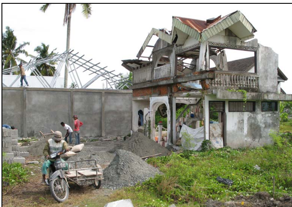
NEW GROUND-FLOOR-ONLY HOUSES ARE BEING BUILT ON OLD FOUNDATIONS
