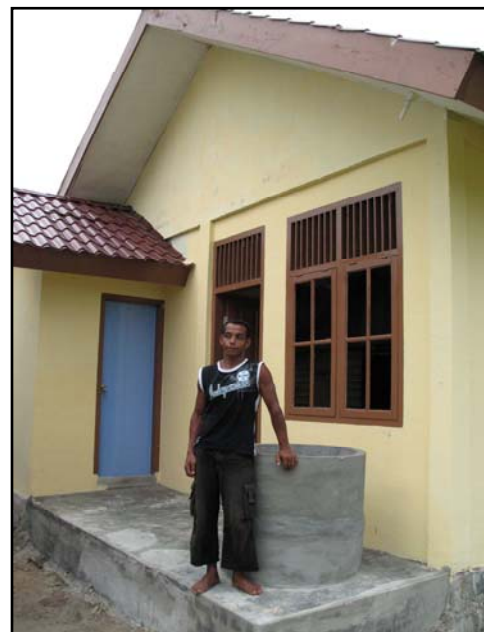
NEW HOUSE WITH NO VENTILATION VENTS UNDER THE ROOF
