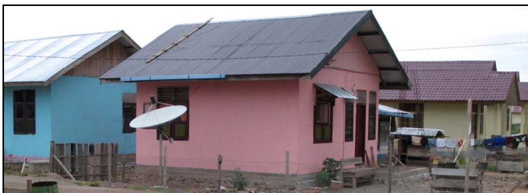
THE OCCUPANT OF THIS HOUSE IS ALREADY ADDING A PORCH
