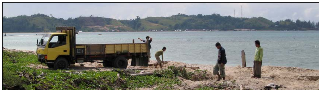
SAND BEING COLLECTED FROM THE SEASHORE – THIS SHOULD NEVER BE USED FOR REINFORCED CONCRETE
