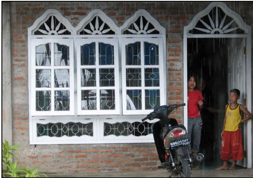
LOW-PLACED VENTILATION WINDOWS CAN BE OPENED WHEN DOOR IS CLOSED
