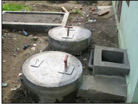
PHOTO LEFT: AN OPEN SEPTIC TANK MADE FROM CONCRETE RINGS. THE FOOTING OF THE RINGS IS ANCHORED TO A WIDER BASE PLATE TO AVOID FLOATING IN HIGH GROUNDWATER AFTER THE TANK IS EMPTIED.
