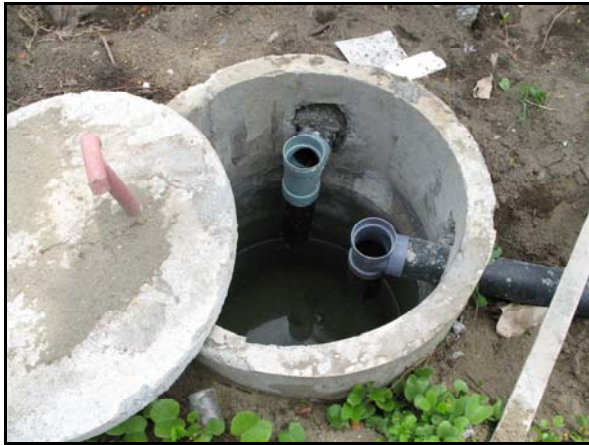
PHOTO LEFT: AN OPEN SEPTIC TANK MADE FROM CONCRETE RINGS. THE FOOTING OF THE RINGS IS ANCHORED TO A WIDER BASE PLATE TO AVOID FLOATING IN HIGH GROUNDWATER AFTER THE TANK IS EMPTIED.
