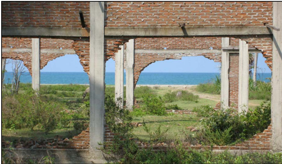
WALLS KNOCKED OUT FROM BETWEEN A SUPPORTING REINFORCED CONCRETE FRAME STRUCTURE
