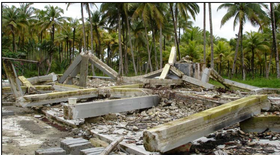
EXAMPLE OF EXCESSIVE FORCES ON NON-ANCHORED INFILL WALLS, COMBINED WITH LACK OF STIRRUPS IN THE MAXIMUM MOMENT AREAS OF THE SUPPORT COLUMNS (PHOTO ALEXANDER ANGERMAIER)
