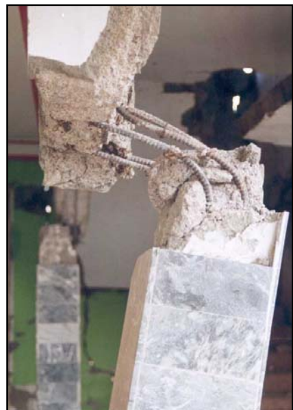
TYPICAL COLUMN FAILURE – NO STIRRUPS
