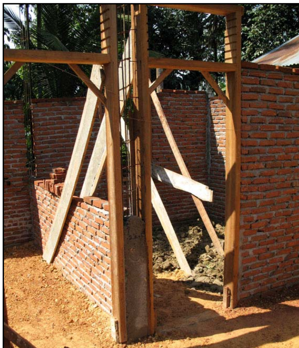
STIFFENER COLUMN CAST BETWEEN TWO DOORS
