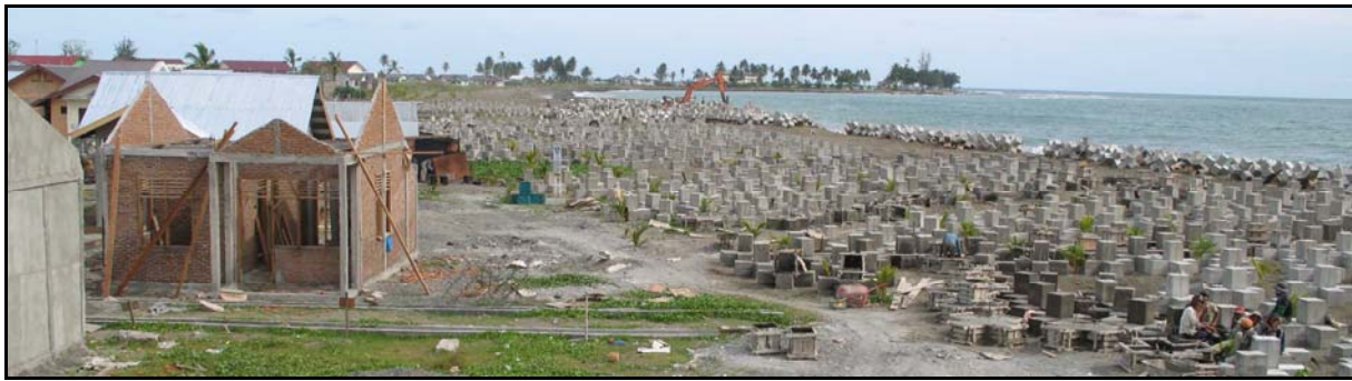
CONCRETE CROSSES CAST ON THE SHORE AND TRANSPORTED TO CREATE AN EROSION CONTROL WALL
