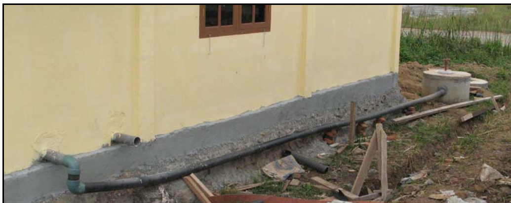
UNCOMPLETED SEWERAGE SYSTEM WITH EXPOSED PVC PIPE FROM TOILET TO SEPTIC TANK AND SOAK AWAY
