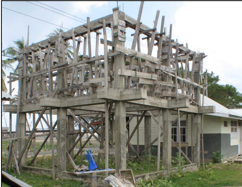
SUPPORTING COLUMN CONSTRUCTION (SPACE-FRAME STRUCTURE)
