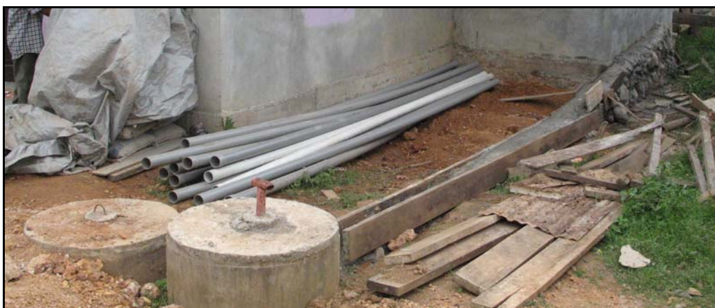
PVC PIPES MASONED IN WITH STONES ALONG THE HOUSE AND CAST INTO CONCRETE FOR PROTECTION
