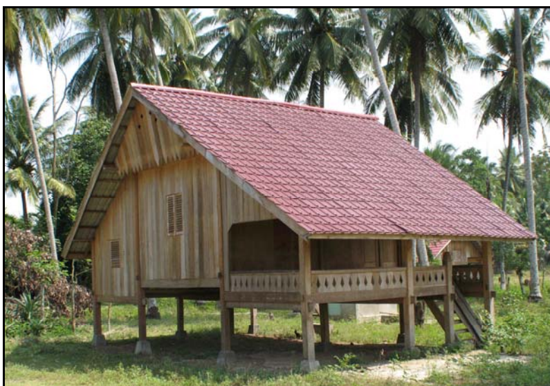
THE FIRST WOODEN HOUSES WERE OFTEN BETTER THAN WHAT THE PEOPLE LOST
