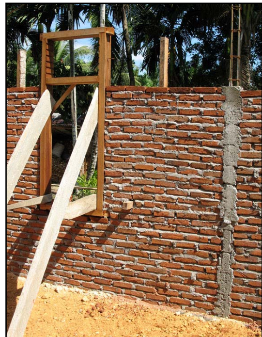
STIFFENER COLUMN CAST IN LONG WALL
