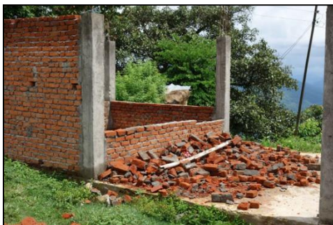
Above (Nepal): no anchors between column and masoned wall caused this wall to collapse.
