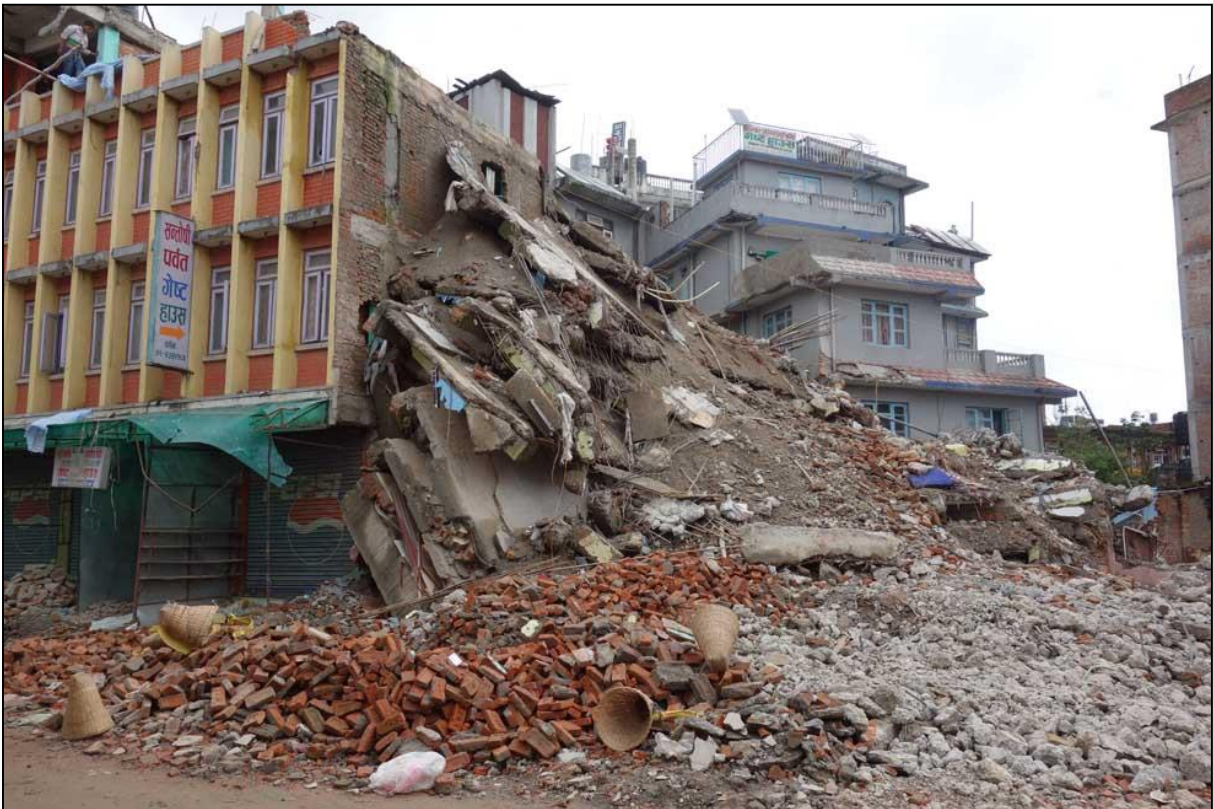
Photo by the Author after the 25 April 2015 earthquake in Kathmandu.
