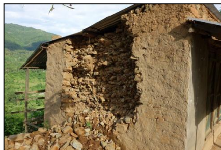
Nepal – rural and urban unreinforced masonry (URM)
