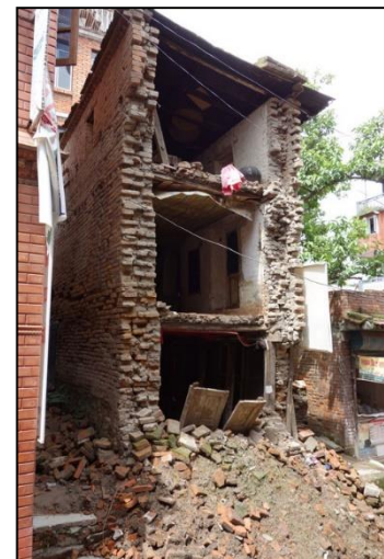
Nepal – rural and urban unreinforced masonry (URM)
