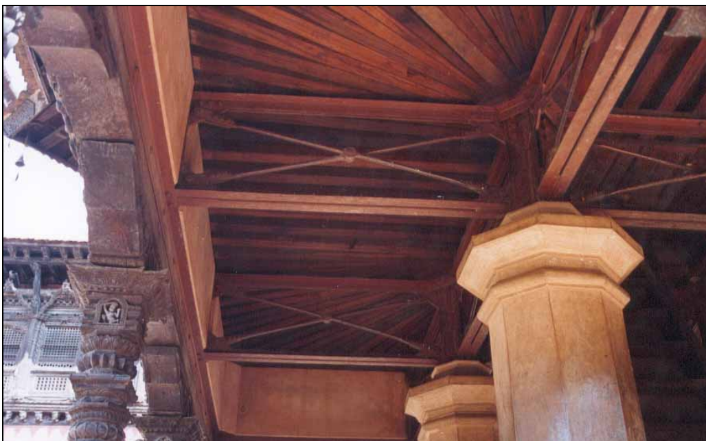
Chyasilin Mandapa Temple in Bhaktapur Durbar Square with internal metal bracing in reconstructed and restored temple.
