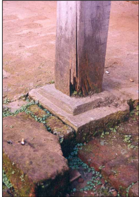
Column with base starting to rot due to up-splashing water.
