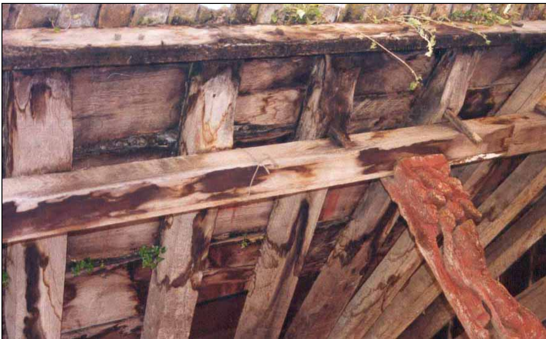
Rotting roof beams and planks as a result of leaking roof and permanent humidity in the soil layer under the roofing tiles.
