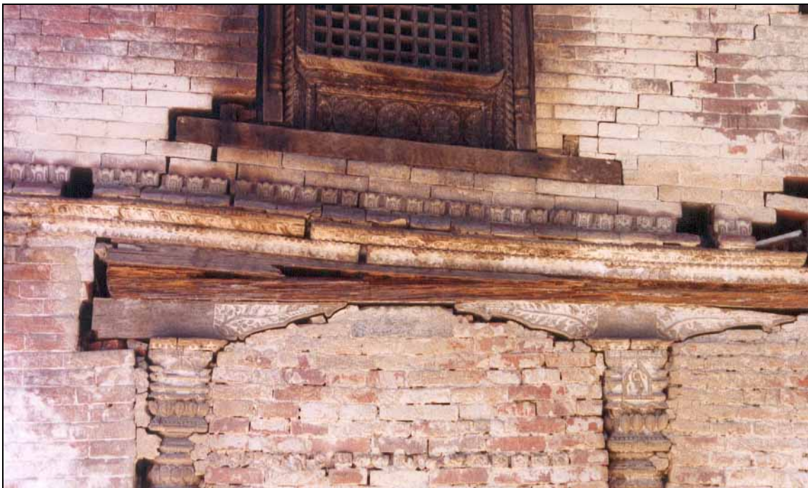
Beam over columns completely pressed flat due to wood rot. Infill walls are made in the window openings to support against collapse.
