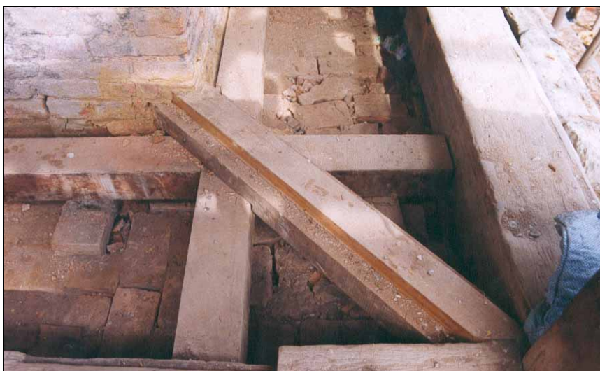
Reconstruction of the Sanctum floor with dovetail connection in the outside beam and half-wood connection for the inner beams. The diagonal beam in the corner supports the floor planks.
