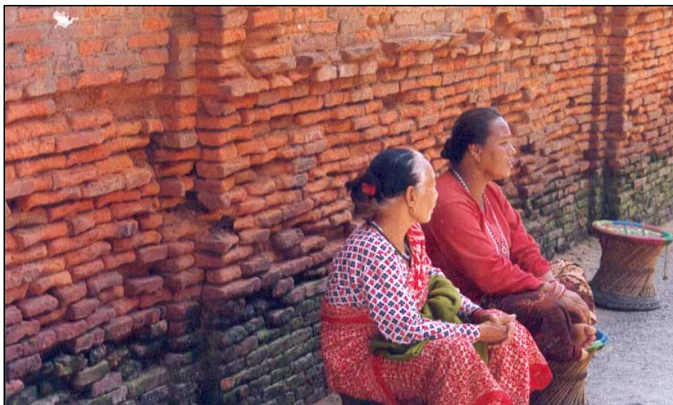
Burned brick wall deteriorated due to rain. Algae growing on lower side due to humidity.
