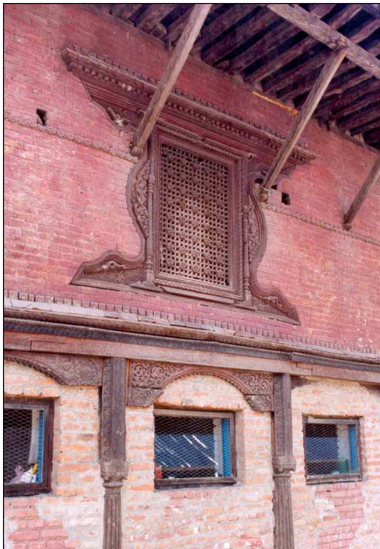
Above the columns and lintel a built-out ridge can be noted. The ridge partly protects the lintel and can hide floor anchorage.
