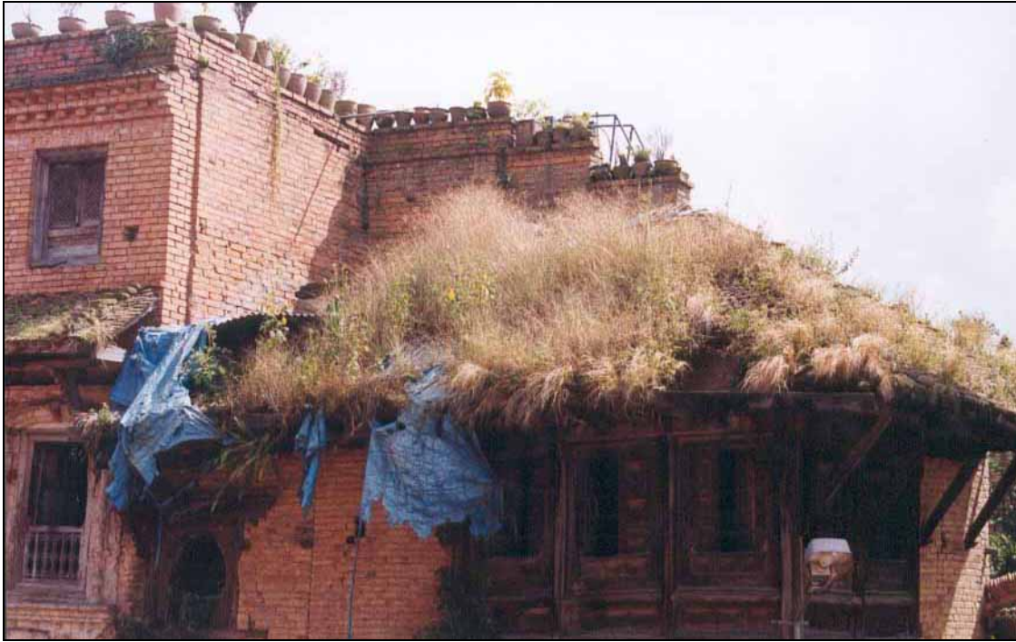
Almost collapsed roof with heavy vegetation.
