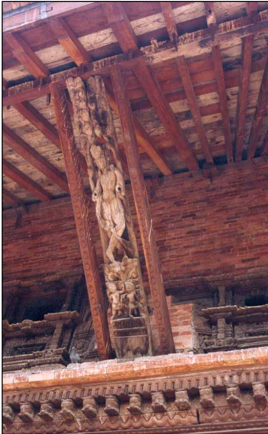
Old carved roof strut supported with two new side supports (left). Bottom of roof strut support repaired with a new piece of wood (right).
