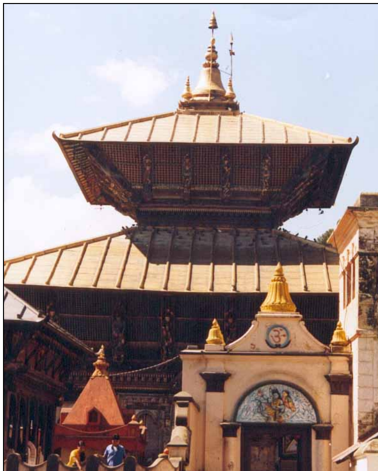
Pashupatinath Temple with a lightweight roof construction with copper plating. This will cause lesser horizontal forces during earthquakes.
