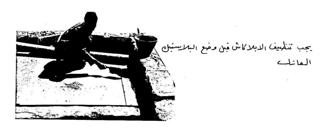
The roof needs carefull cleaning. no gravel or nails should damage the roofing plastic.
