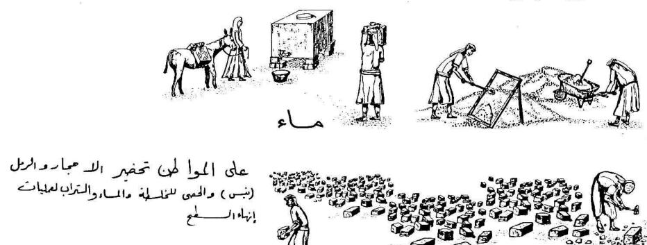
The beneficiary will prepare the stones, sand for masonry, gravel for concrete and water and soil for the roof.
