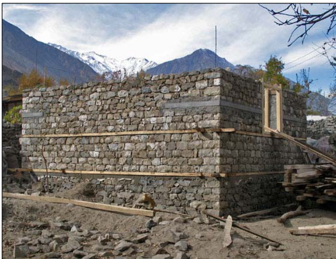
Left: House 2 – the floor is at the level of the first timber line; entrance door is at the rear. Right: Insulating plaster layer at the window opening.
