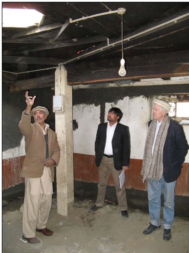
Traditional Pamiri houses have low vulnerability for earthquakes, but when retrofitting, the roof should be made lighter and thermal insulation applied, including a roof hatch window.
