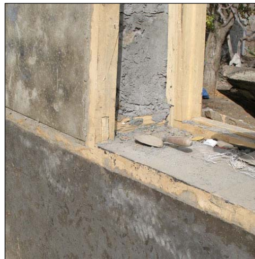
Left: House 2 – the floor is at the level of the first timber line; entrance door is at the rear. Right: Insulating plaster layer at the window opening.
