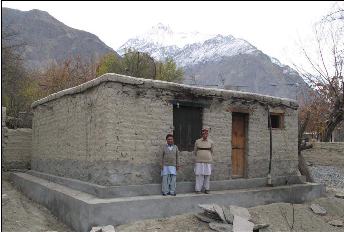
View of the massive foundation ring beam of the small one-floor-only adobe house
