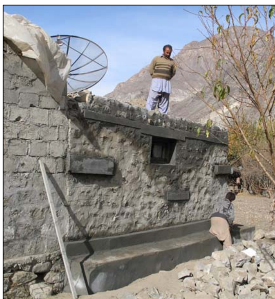
Left: Outside wall of the main room with foundation ring beam and wall stitches.
