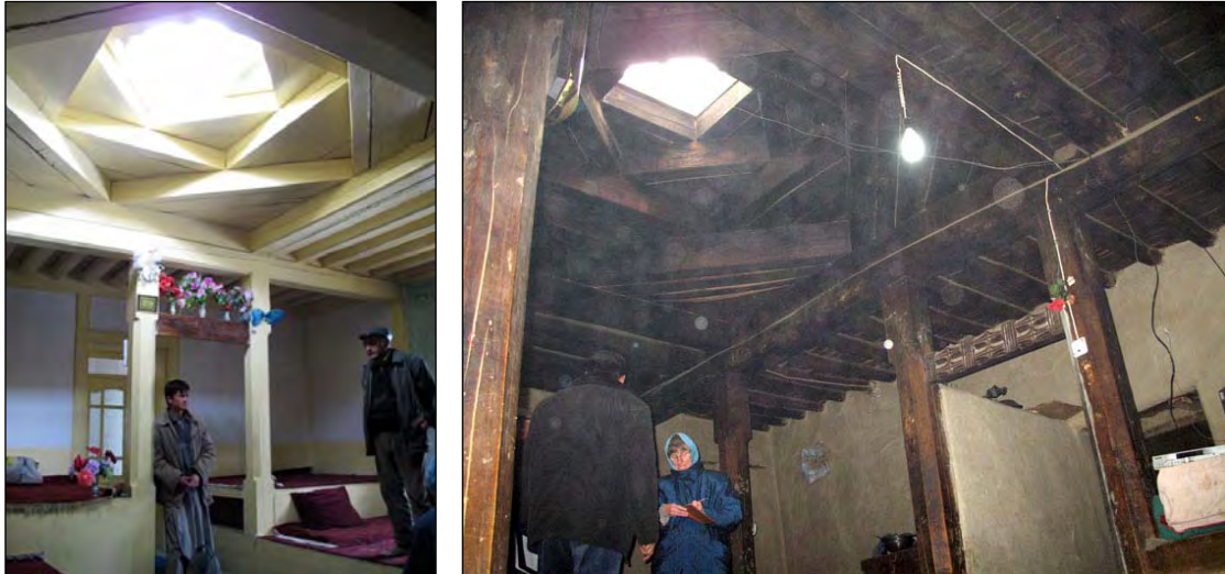
Depending on the age of the Pamiri houses, the roof-to-wall connections are different because in the more recent houses, fewer and thinner supporting timber is used.
