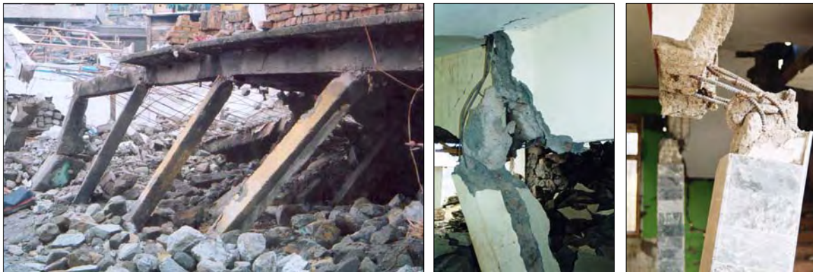
Reinforced concrete constructions are typically heavy and brittle designs that collapse instantly when the earthquake forces exceed the construction design. The reinforcement does not hold the broken concrete together. At the maximum moment area, a large number of stirrups are needed to avoid sudden collapse.
