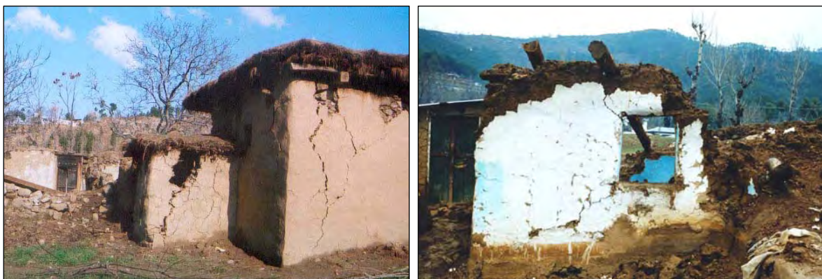
Most adobe houses will fail during an earthquake, even when not located near the epicentre.
