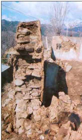
Left photo: Shows the loose bondage in the clay masoned rubble stone wall.
