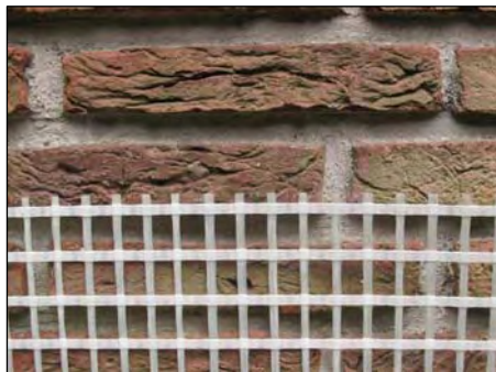
VITRULAN Panzer Openings 12 mm x 20 mm 1000kg/10 cm stress resistance
