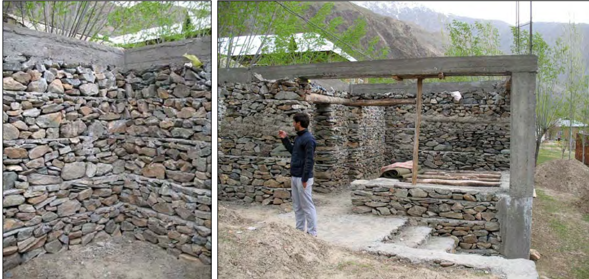
On the outside corner of the left photo, a linking column of 45 cm x 45 cm section joins the walls. The right-hand photo is the same building, showing the much lower field level.
