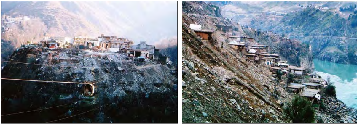
In the Kashmir earthquake nearly all buildings that were constructed on slopes of more than 30% collapsed. The remaining lightweight one-floor timber houses were severely damaged.
