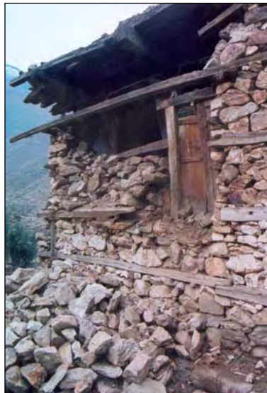
Left photo: Shows the loose bondage in the clay masoned rubble stone wall.
