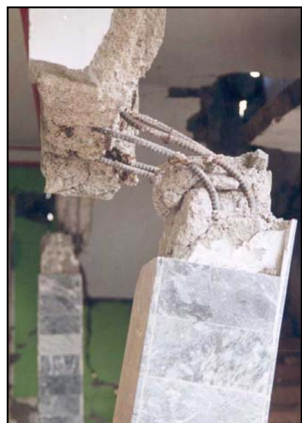
Typical Column Failure – No Stirrups
