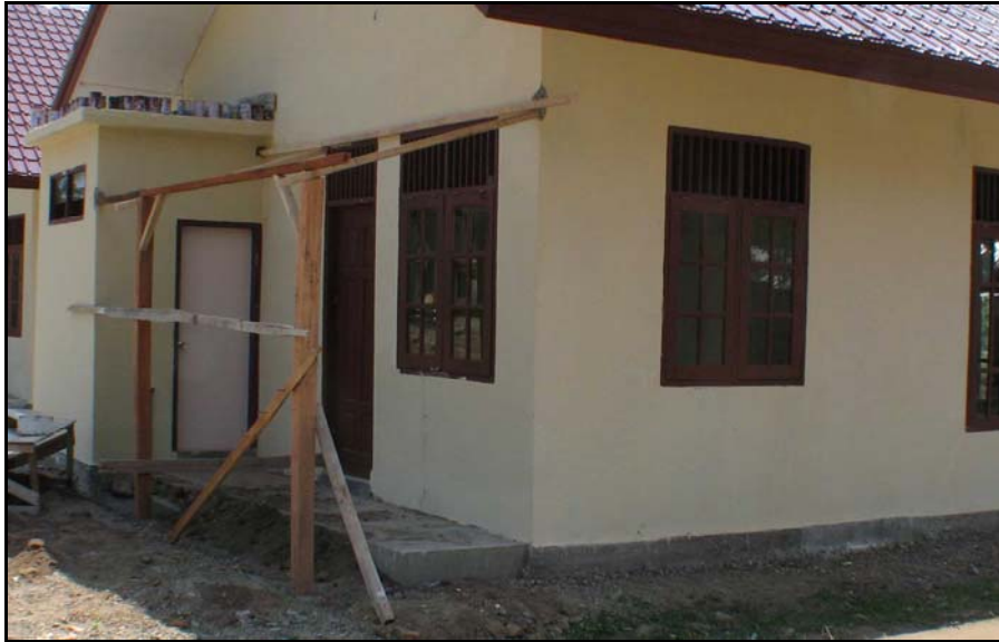
Kitchen Extension at Rear of House
