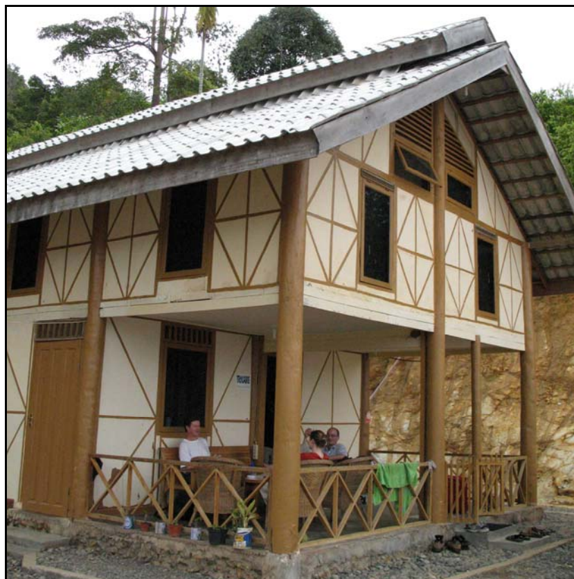
TWO-STOREY DEMONSTRATION HOUSE WITH WOODEN FRAMEWORK, INFILLED WITH COCONUT-FIBRE PLASTERED WALLS AND A MCR TILE ROOF. THE BUILDING IS USED BY CARITAS CZECH AS A FIELD OFFICE AND ACCOMMODATION.
