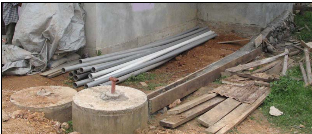
PVC PIPES MASONED IN WITH STONES ALONG THE HOUSE AND CAST INTO CEMENT FOR PROTECTION
