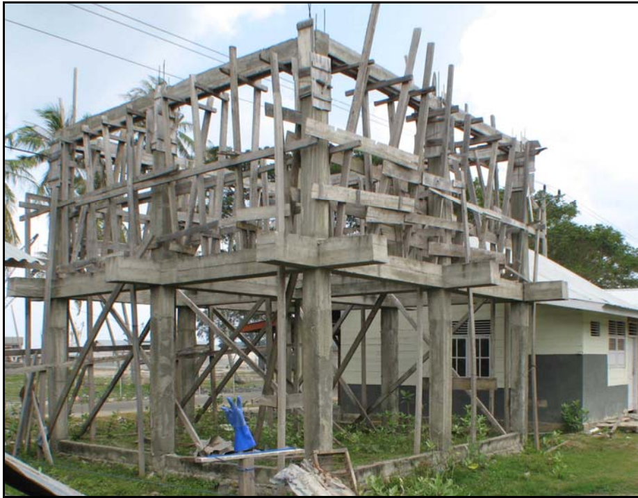
SUPPORTING COLUMN CONSTRUCTION (SPACE-FRAME STRUCTURE)
