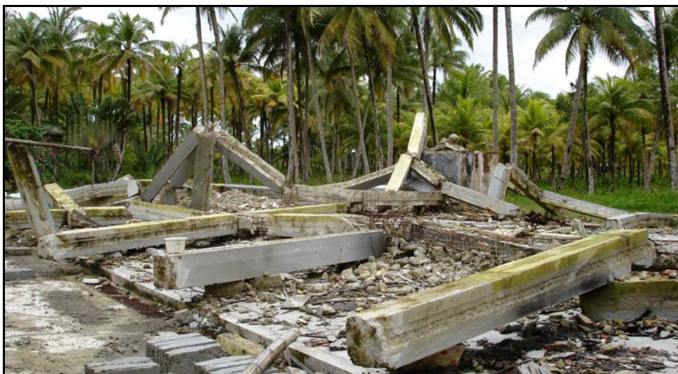
EXAMPLE OF EXCESSIVE FORCES ON NON-ANCHORED INFILL WALLS, COMBINED WITH LACK OF STIRRUPS IN THE MAXIMUM MOMENT AREAS OF THE SUPPORT COLUMNS
