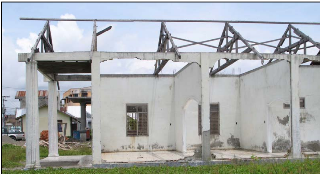
WALLS KNOCKED OUT FROM BETWEEN A SUPPORTING REINFORCED CONCRETE FRAME STRUCTURE
