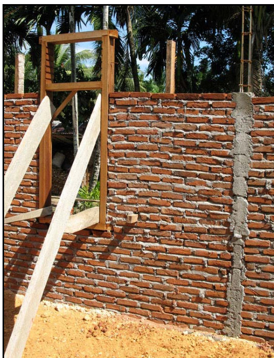
Stiffener Column Cast
