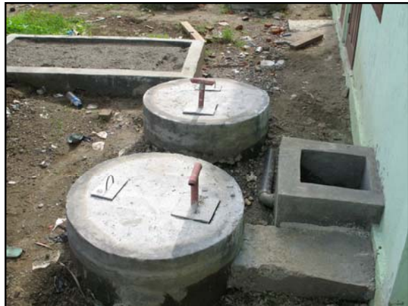
Photo Left: An open septic tank made from concrete rings. The foot of the rings is widened to avoid floating in high groundwater level.
