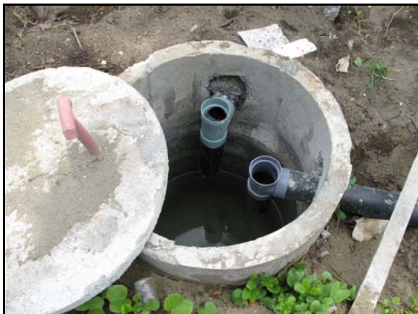
Photo Left: An open septic tank made from concrete rings. The foot of the rings is widened to avoid floating in high groundwater level.
