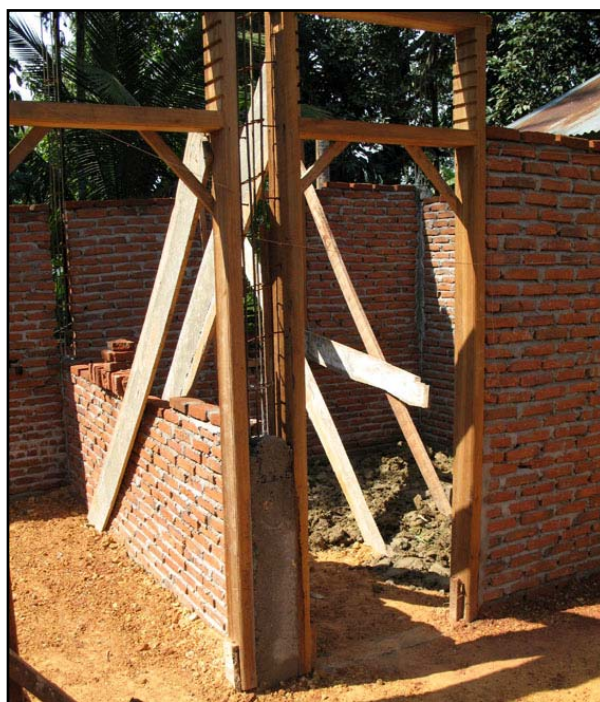
Stiffener Column between Two Doors
